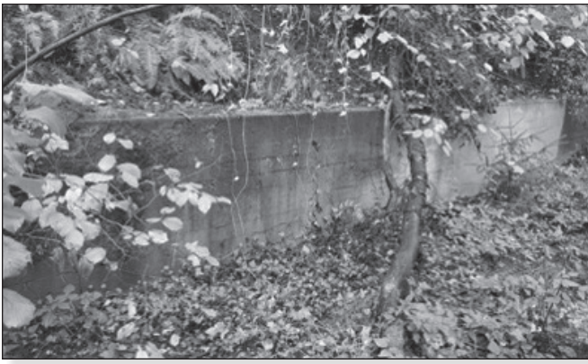
The century-old concrete wall along the former tennis court
